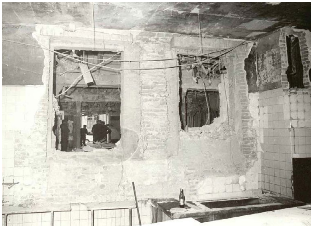
Internal view of Tobogán showing damage at its adjoining wall with Rolando.
