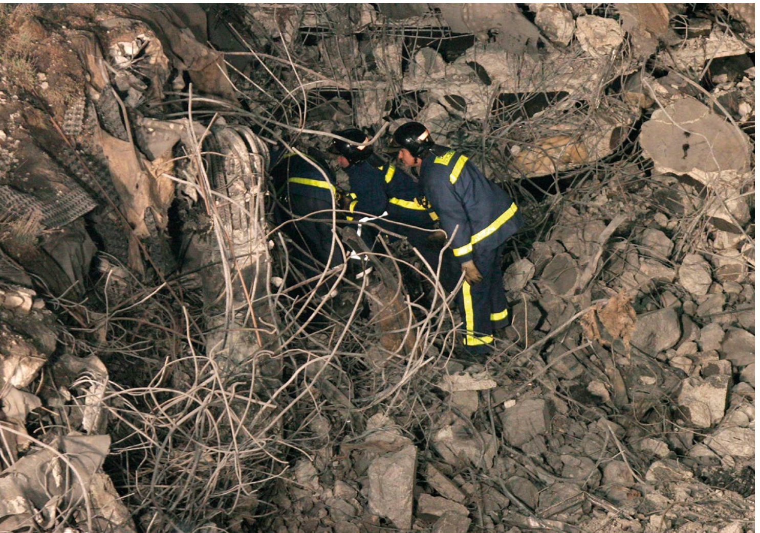
Fig. 6. A group of firefighters inspect the rubble of the car park at terminal T4 of Madrid's Barajas airport, destroyed by an ETA bomb, in their search for two missing people (02/01/2007). Source: Alberto Martín, EFE
